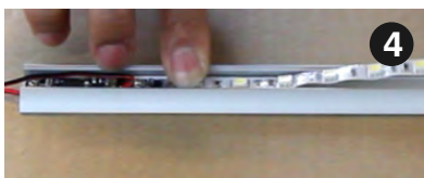
4 Lay the LED strip light down on to the insulating double sided tape
